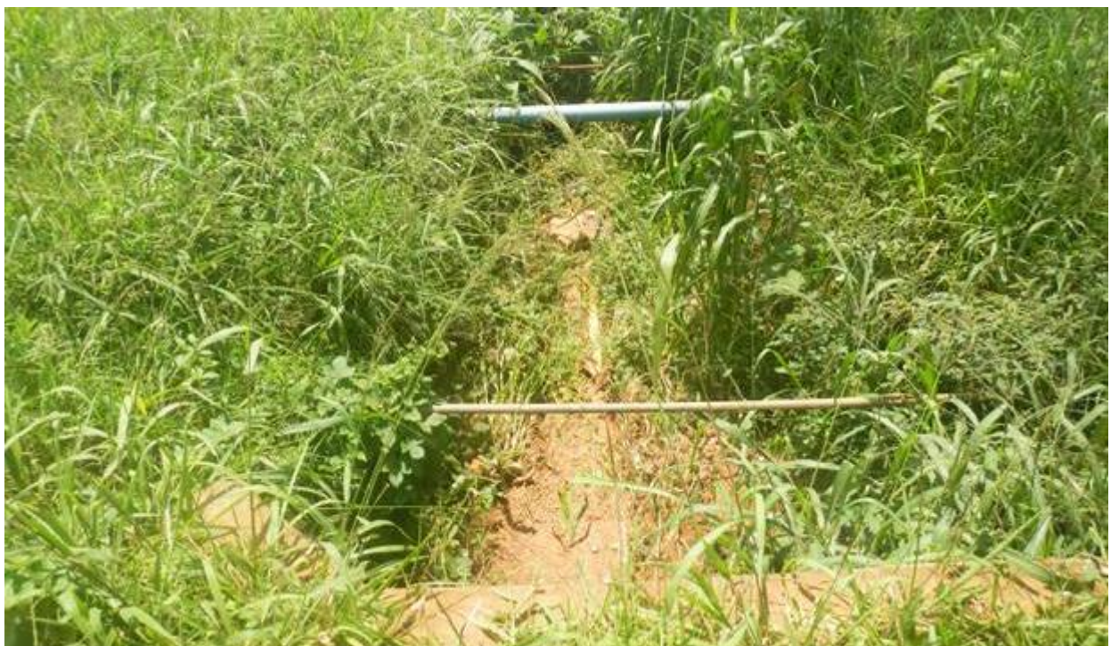
Photo 4.1: Drainage channel with water supply lines running from Butabika Hospital and through the proposed site
