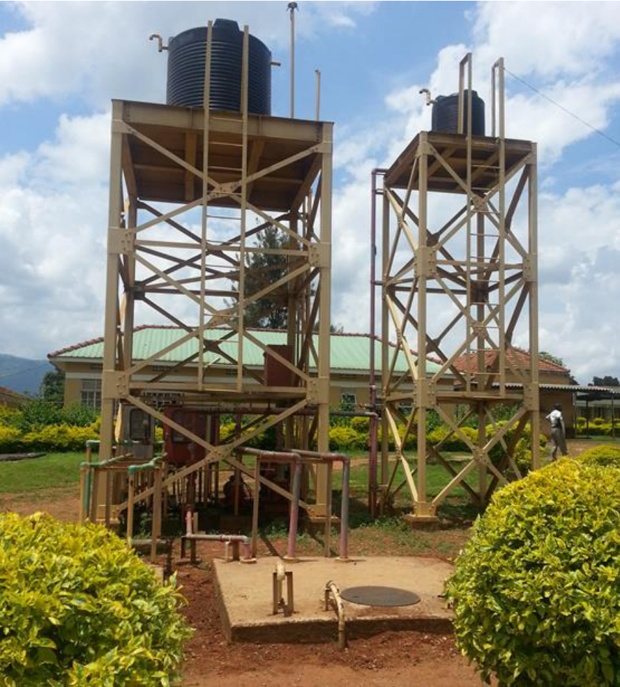
Photo 4.7: Groundwater supply system for emergency water supply to the ward of expectant mothers
