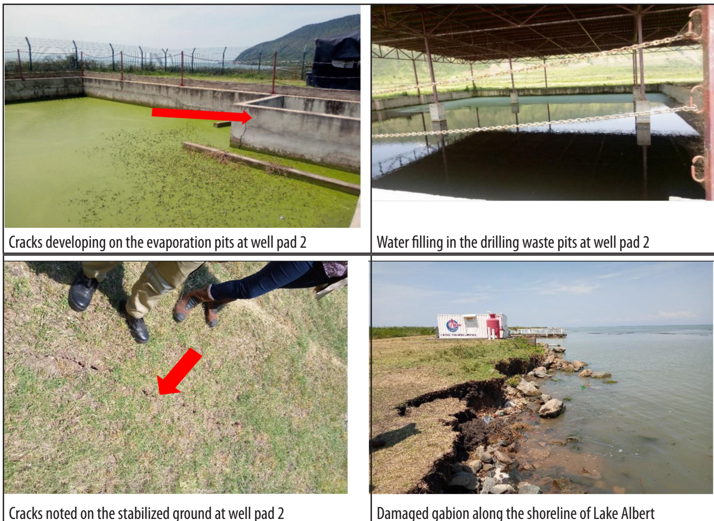
Figure 14: Images of cracks, bunding and damaged gabion during inspection of Tilenga and Kingfisher projects. Source: PAU, 2020
