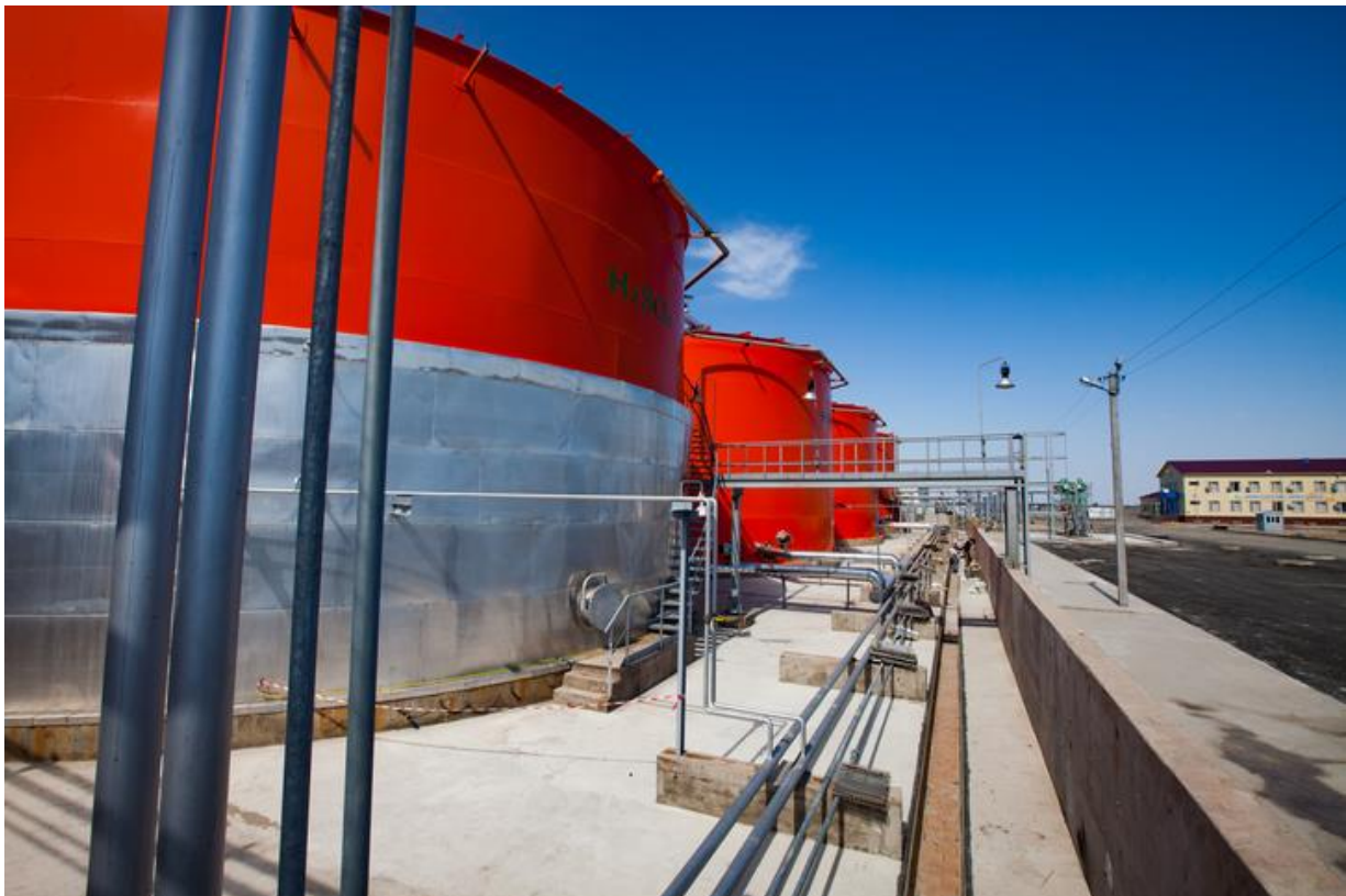
Figure 38: Fully bunded Sulfuric Acid Storage Tanks will be in place at Makuutu
