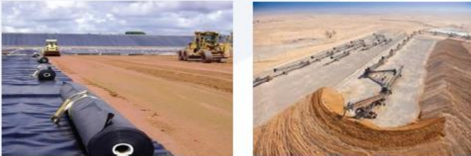
Figure 3: Heap leach construction, showing the plastic liner being laid on the left. On the right, the base is applied on top of the liner and the ore is stacked on top within the heap leach cells
