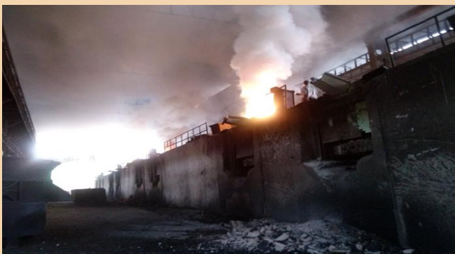
An image showing indoor Air Pollution at Iganga Steel Division
