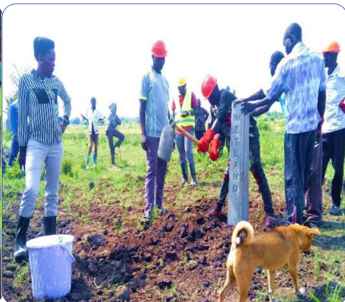
Figure 2.1.18: The technical team working with the local community to install a precast concrete pillar at Amese village adjacent to Kamurojo wetland
