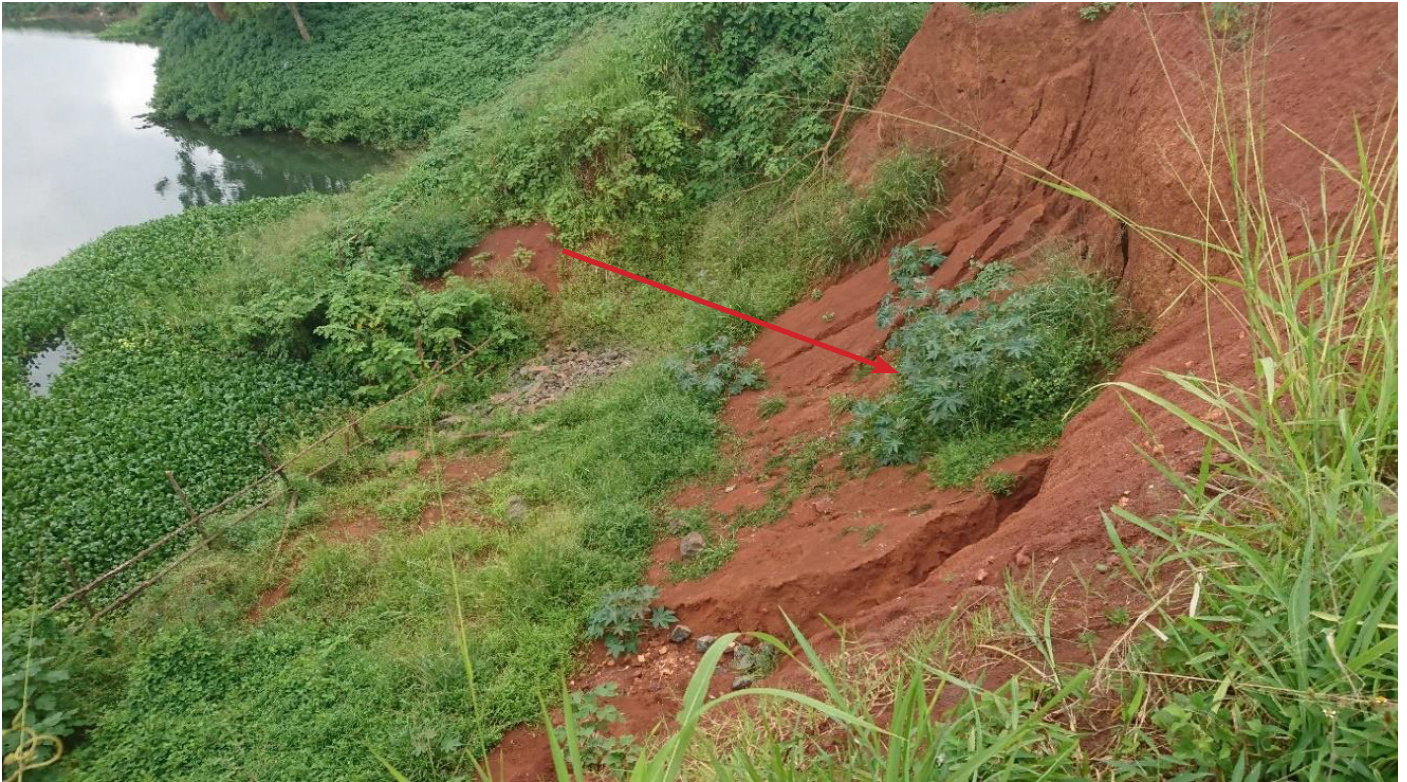
Figure 2.1.1: Section of collapsed slope along the left bank of the reservoir of Bujagali Hydropower Plant.
